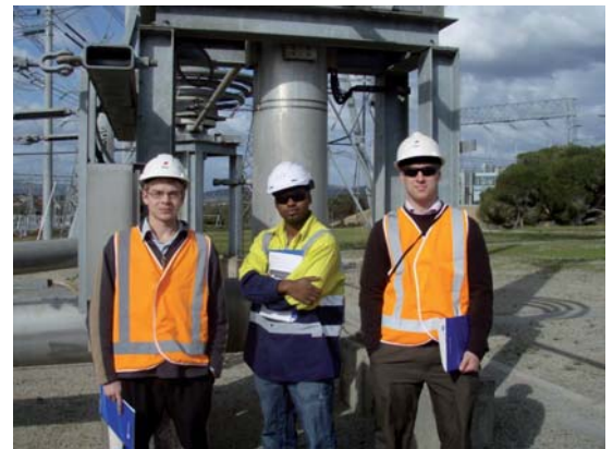
Tenix Engineers (from Left), Terry Williamson, Dilogen Emmanuel and Kieran Robson-Garth standing in front of one of the 500kV SF6 line terminations
